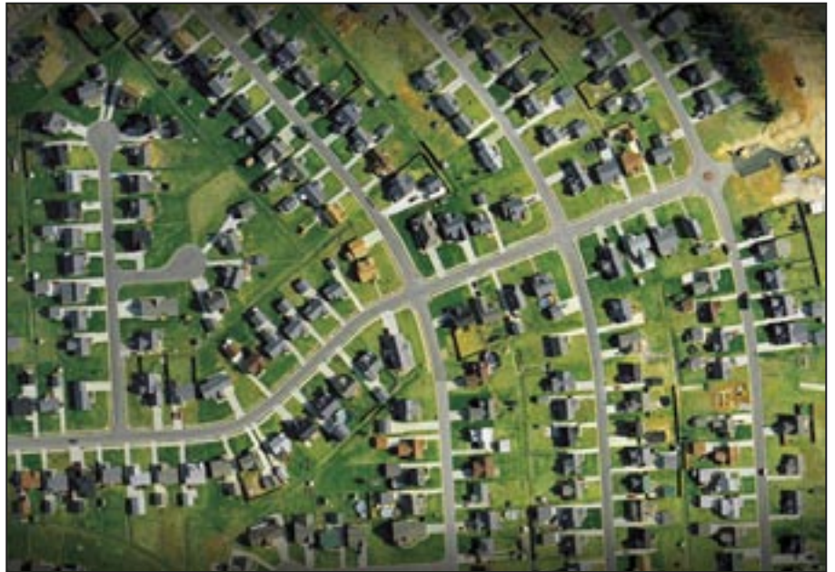
Aerial view of Heritage Creek.
