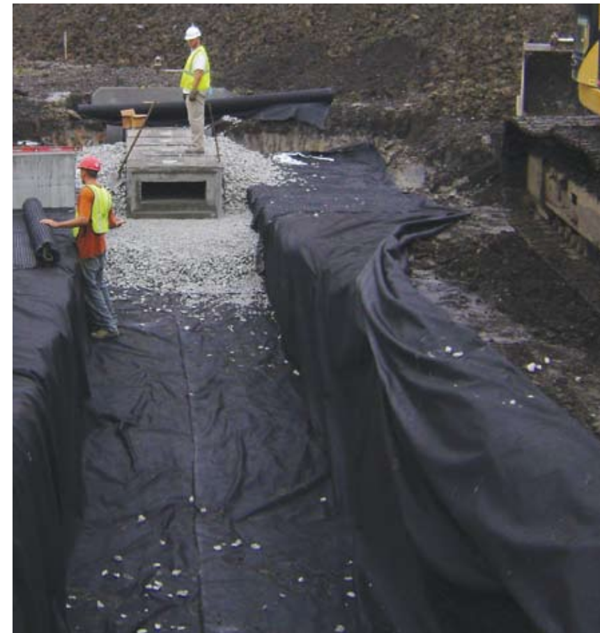
Installing drainage pipe as part of the Crittenden Drive Relocation Project.
