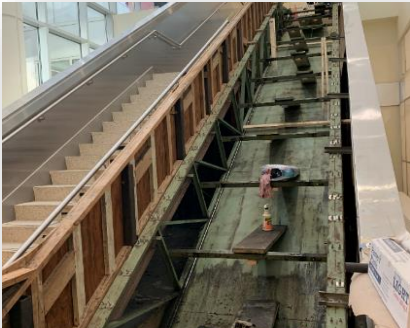
Elevator, Escalator Replacement
