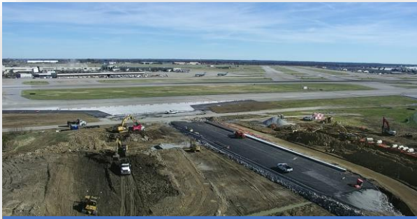
Northwest Quad Development / Taxiway A Connector
