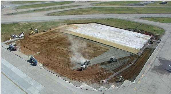
Geothermal Wellfield and Terminal Apron Construction
