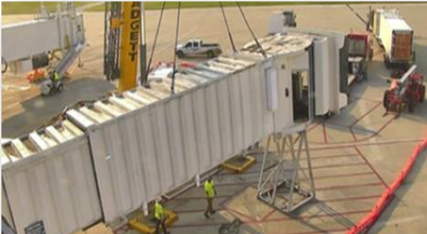
Replacement of Terminal Passenger Boarding Bridges
