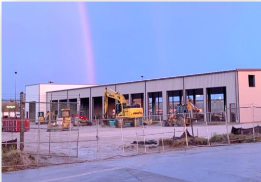
New Snow Removal Equipment Storage Facility
