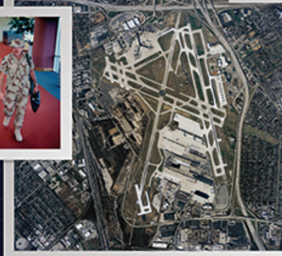
Beginning Construction of Runway 17/35L (West Runway)
