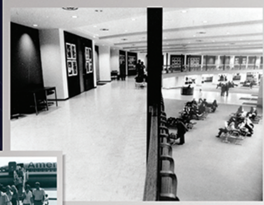
Newly Expanded Lee Terminal
