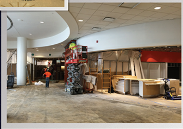
Construction of the TODAY Store
