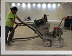
Terrazo floor installation
