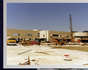
Exterior Construction of the New Terminal
