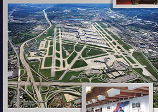
SDF Airfield Overview
