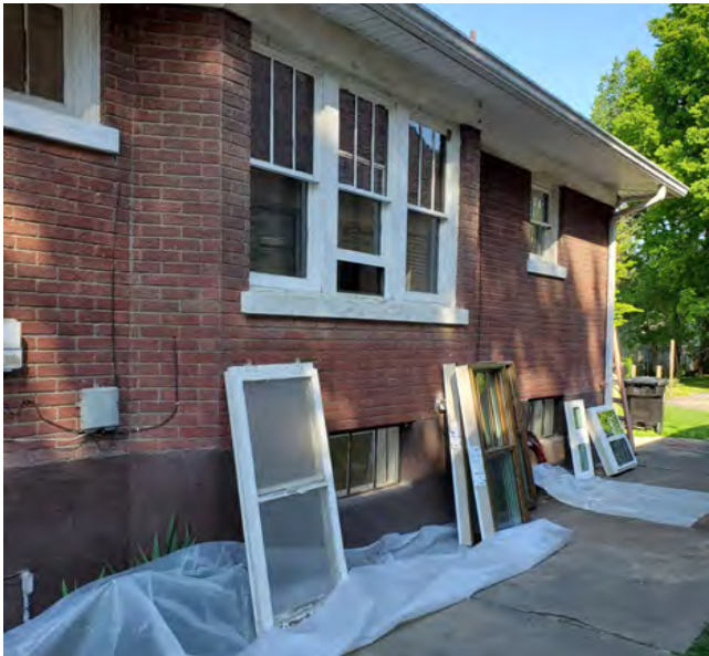
Window replacement for sound installation
